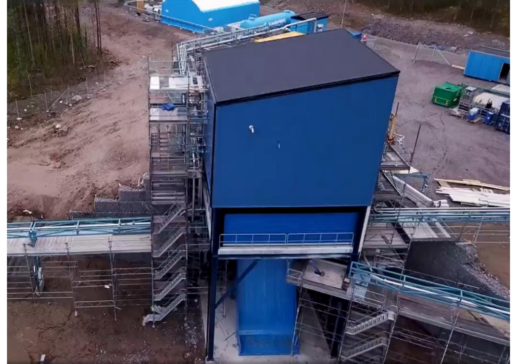
ISAR Test Site
